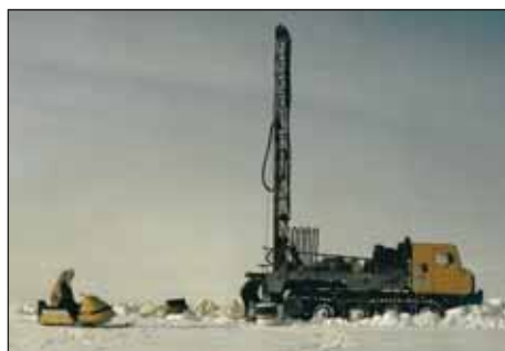
A seismic shot hole drill operates on the tundra during seismic surveys on the North Slope in the early 1960s.
