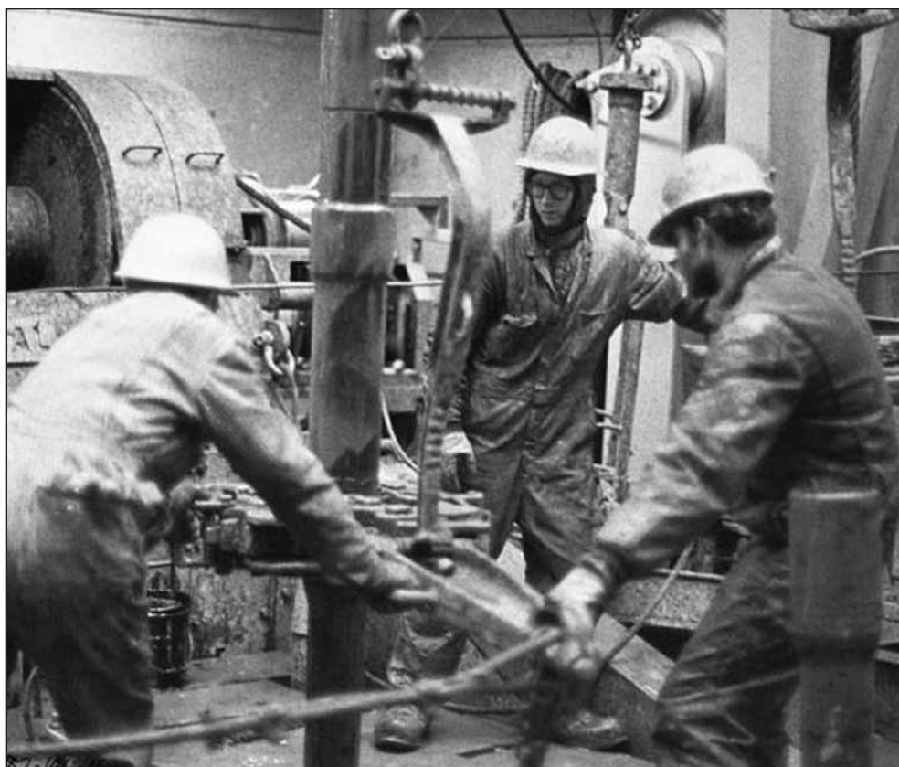
Drilling rig crews have played a vital role in development of the giant Prudhoe Bay oil field throughout its 40-year history. Here roughnecks connect pipe string during delineation drilling at Prudhoe Bay in 1969. Extreme weather conditions in the Arctic mandate that the drill floor be enclosed and heated.
